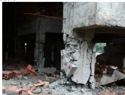
(c) 错层造成短柱剪切破坏
