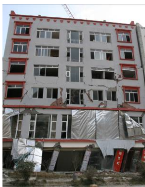
(a) 北川某底框住宅底层严重倾斜破坏 (a) Large story drift at the first story
