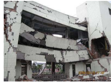
The damage of an office building using horizontal hybrid structure
