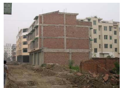
Undamaged masonry structures with concrete structural columns and ring beams in Anxian
