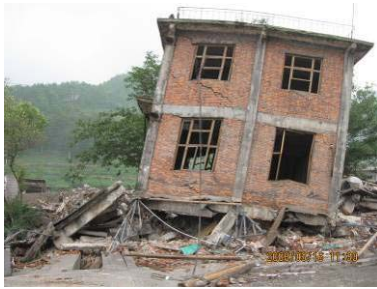
A gas station using masonry structure with bottom RC frame, Hongbai
